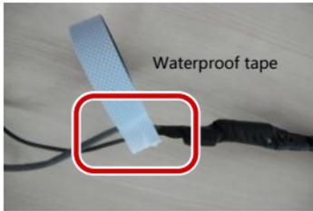
6. Protect the tail cables using waterproof tapes.
